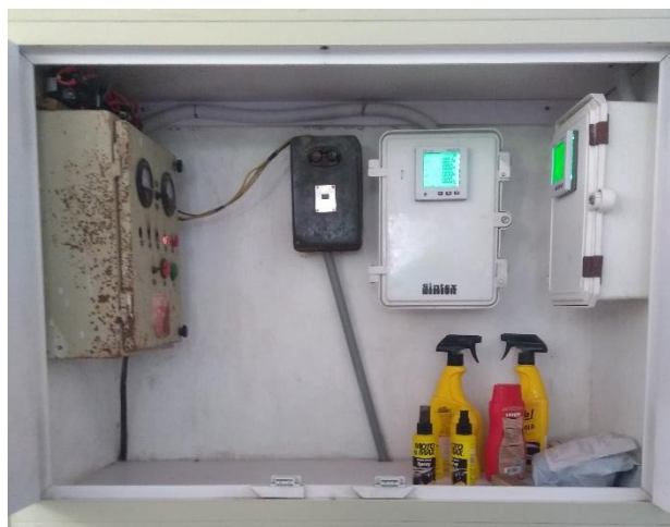
Figure 16 Installation of community level monitoring
