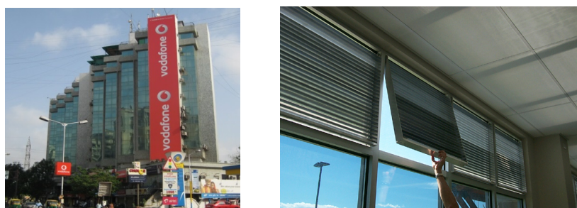
Figure 3: (a) Typical Indian office with no daylight redirection device (b) LightLouver units in clerestory to reflect sunlight into the ceiling
