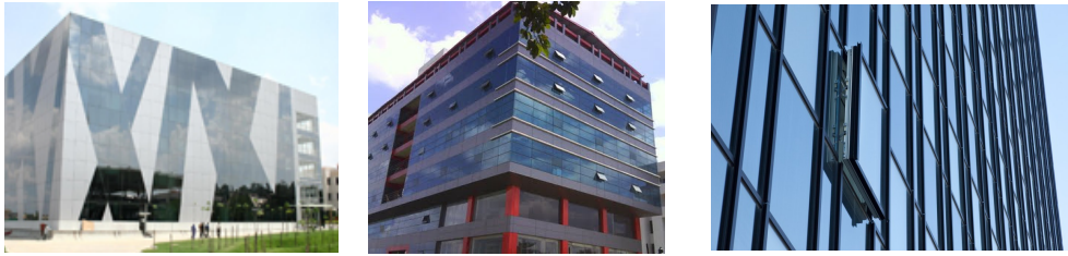
Figure 6: a) Infosys, Bangalore with no operable windows, b) 3i Innfotech EPIP Whitefiled with a modest percent of operable windows, but dark glass c) Deutsche Bank, Frankfurt with high Tvis pop-out windows.
