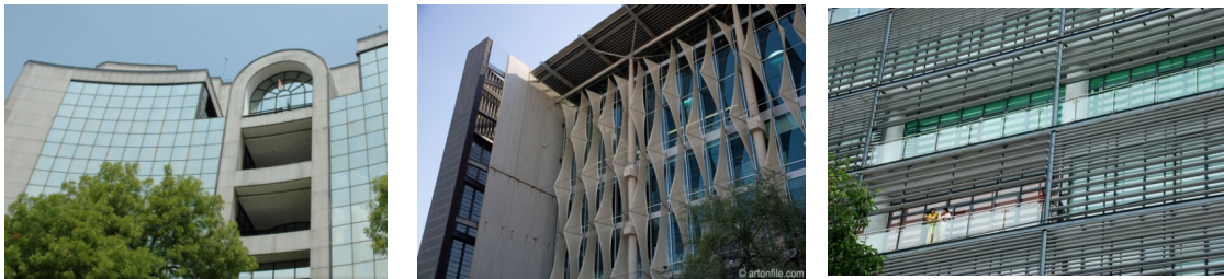
Figure 5: a) DLF Center, Delhi with no shading devices vs. b) vertical awnings on the north face of the Phoenix library, and c) horizontal louvers on south face of Stecalite, Noida.
