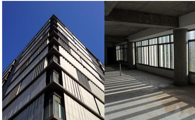
Fig 1: Exterior and interior view of the primary case study, Safal Profitare, Ahmedabad, India.
