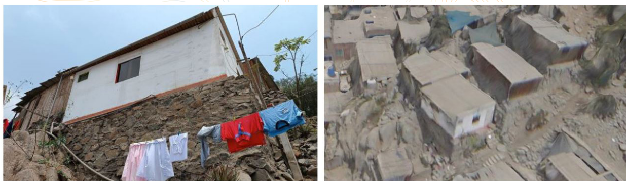
Figure 1: Case study house. Onsite photo (left), 3D reality image from drone survey (right).
