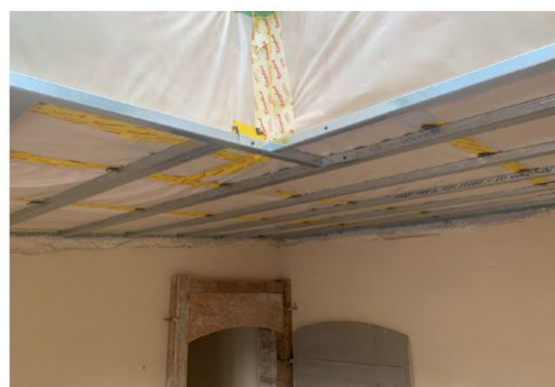
Figure 10: Installation of roof insulation (18 cm mineral wool)
