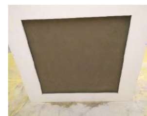
Figure 4: Inner 15mm plaster in cement
