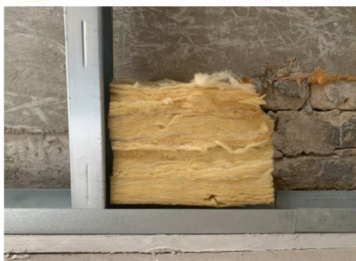
Figure 8: Photo of installation of wall insulation from interior side
