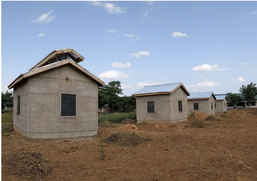
Figure 1: The four experimental buildings (test cells) in Tamale, Ghana. The nearest building has a ridge ventilator.
