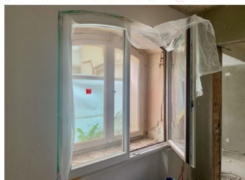
Figure 9: Photo of window enhancements
